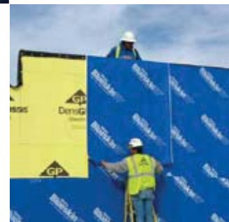
Self-adhered membrane eliminates fasteners that leave holes in the building envelope.
