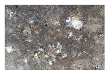
Acidic droppings: A bird on the roof is sure to leave droppings everywhere. Birds have highly acidic droppings that can damage asphalt roofing materials and potentially other equipment on the roof, such as HVAC units. Further, the droppings may stimulate the growth of algae or moss by providing nutrients. Thus, your roof may have a shorter life span if it is exposed to bird droppings.
